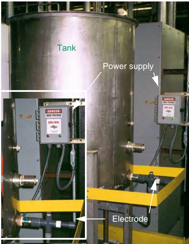
Figure 2: Installation of the Zeta Rod electrode and power supply at the shear spray lubricant mixing tank.
