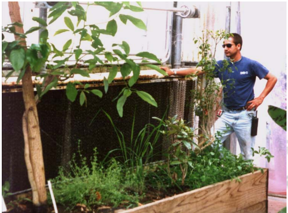
Figure 1: The greenhouse climate wall at Biosphere 2 Center humidifies and cools interior spaces during Arizona’s hot, dry climate.
