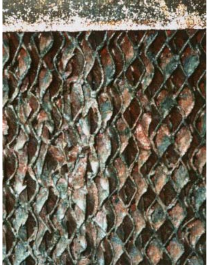
Figure 2: Photos of evaporative cooling media. LEFT (BEFORE Zeta Rod installation) - Significant build-up of slime and scale interferes with wetting of media and impedes air flow. RIGHT - 6 weeks after installation of the Zeta Rod system, layers of fouling and scale swelled and loosened, and the media was restored to clean condition by washing with a low-pressure garden hose.
