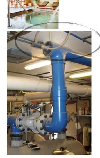
MUNICIPAL SWIMMING POOL: Zeta Rod installed in 6" PVC piping has been continuously treating 220,000 gallons of recirculating municipal pool water in the Arizona desert since 2002.
