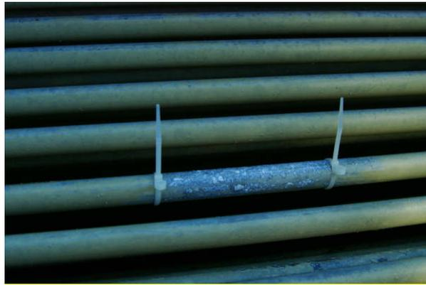
Figure 13. Mechanically cleaned section of upper tubes on the evaporative condenser at Zeta demonstration site (Davis Monthan AFB Fitness Center, July 2007).
