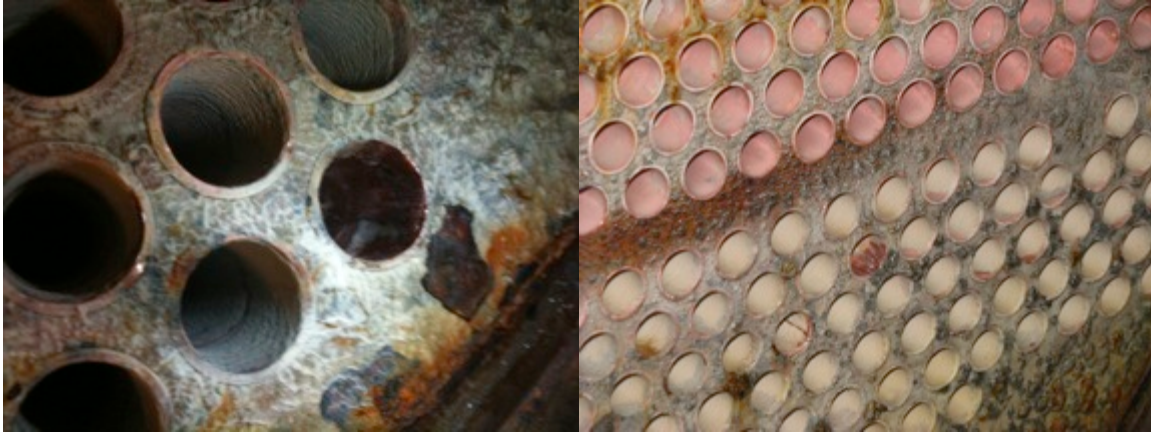
Figure 8: Ft Irwin Bldg 273 (Ctrl) condenser tubes. Feb 2010 (left) scale can be seen on the tube surfaces, a section of one of the tubes was mechanically cleaned to show the copper surface free of scale. Jan 2011 (right) shows the condenser tubes with scale more visible on the second pass of the heat exchanger (lower half) after the condenser ran for approximately 90 days with no treatment and at low cycles of concentration. The outermost section of the tube in the middle was mechanically cleaned to show the copper surface without scale.
