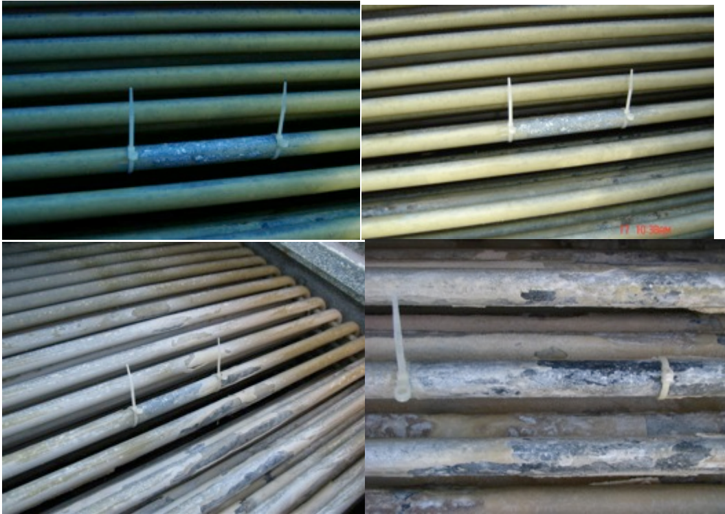
Figure 5: Time progression of Evaporative Condenser Tubes in Test (Bldg 2301) unit at Davis Monthan AFB. Dates pictures were taken (clockwise from upper left) Sept 2007, June 2008, March 09, March 2011
