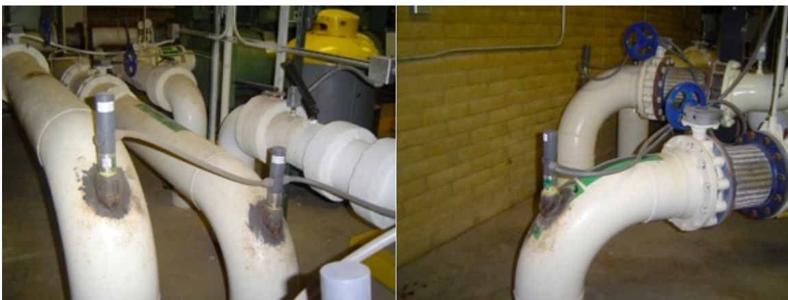
Figure 4: Zeta Rod electrodes mounted on 1 1/2" thread-o-let fitting in cws & cwr lines at Fort Huachuca SCP.
