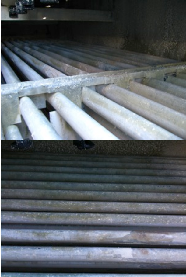
Figure 6: General condition of the tubes at Davis Monthan Bldg 2301 after 44 months of operating at an average of 5 cycles of concentration with no chemicals (March 2011)
