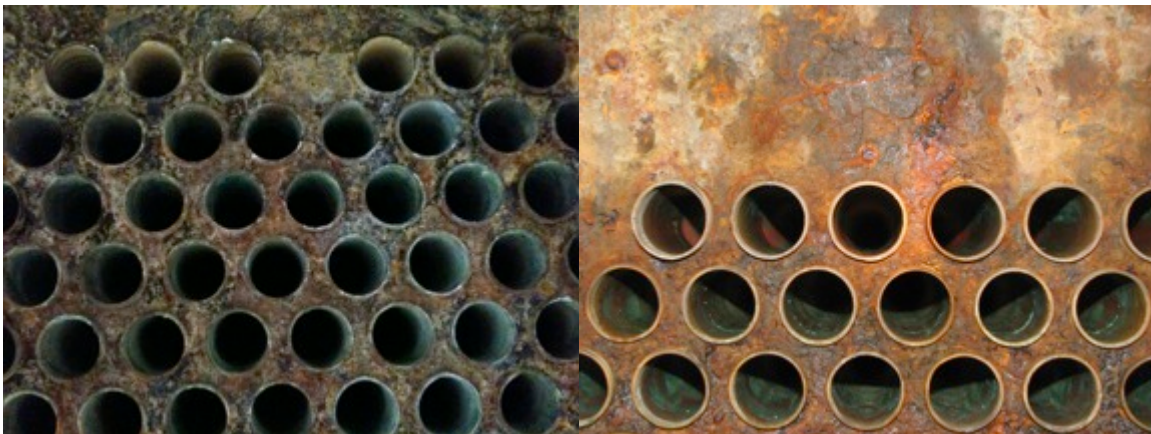
Figure 7: Ft Irwin Bldg 263 (test) condenser tubes during Borescope inspections Feb 2010 (left) and Jan 2011 (right),
